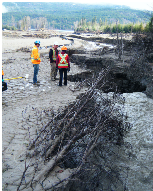
Slope instability and red tailings deposited within the Hazeltine Creek channel (September 22, 2014).
