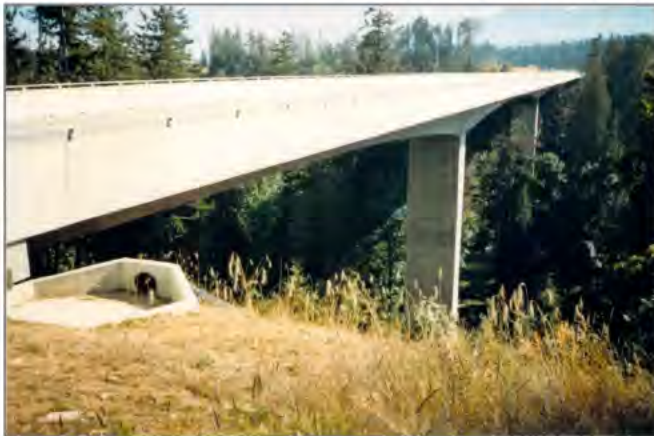
FIGURE 4-3. EXAMPLE OF BOX GIRDER-TYPE STRUCTURE OVER THE TSABLE RIVER
